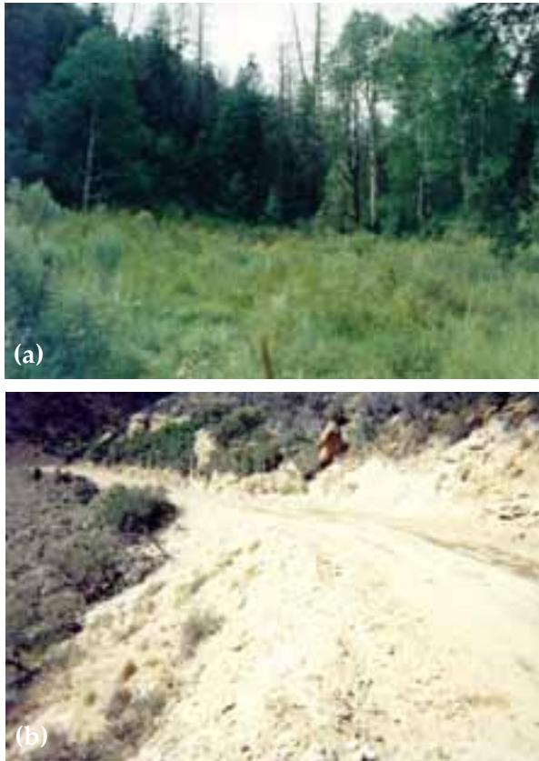
Figure 4. (a) Trap location in Little Berry Canyon on the East Tavaputs Plateau, Utah. (b) Improved road in Horse Canyon to permit passage of semi-tractors and drilling rig. Prior to construction this road was passable only by high-clearance, 4-WD vehicles.
