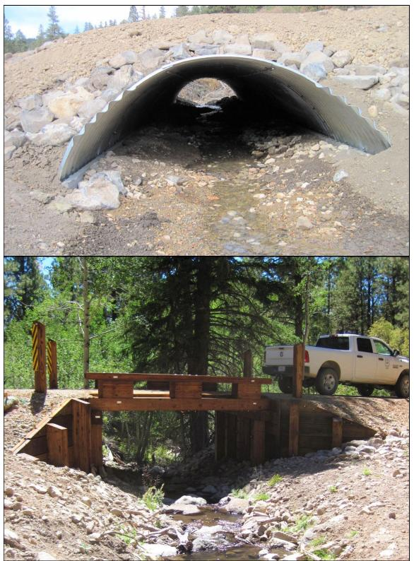
Figure 6. Fish-passable culvert (top) and timber crib bridge (bottom) that replaced previously impassable culverts in Hall Creek at Forest Highway 17 and the upper administrative road, respectively.
