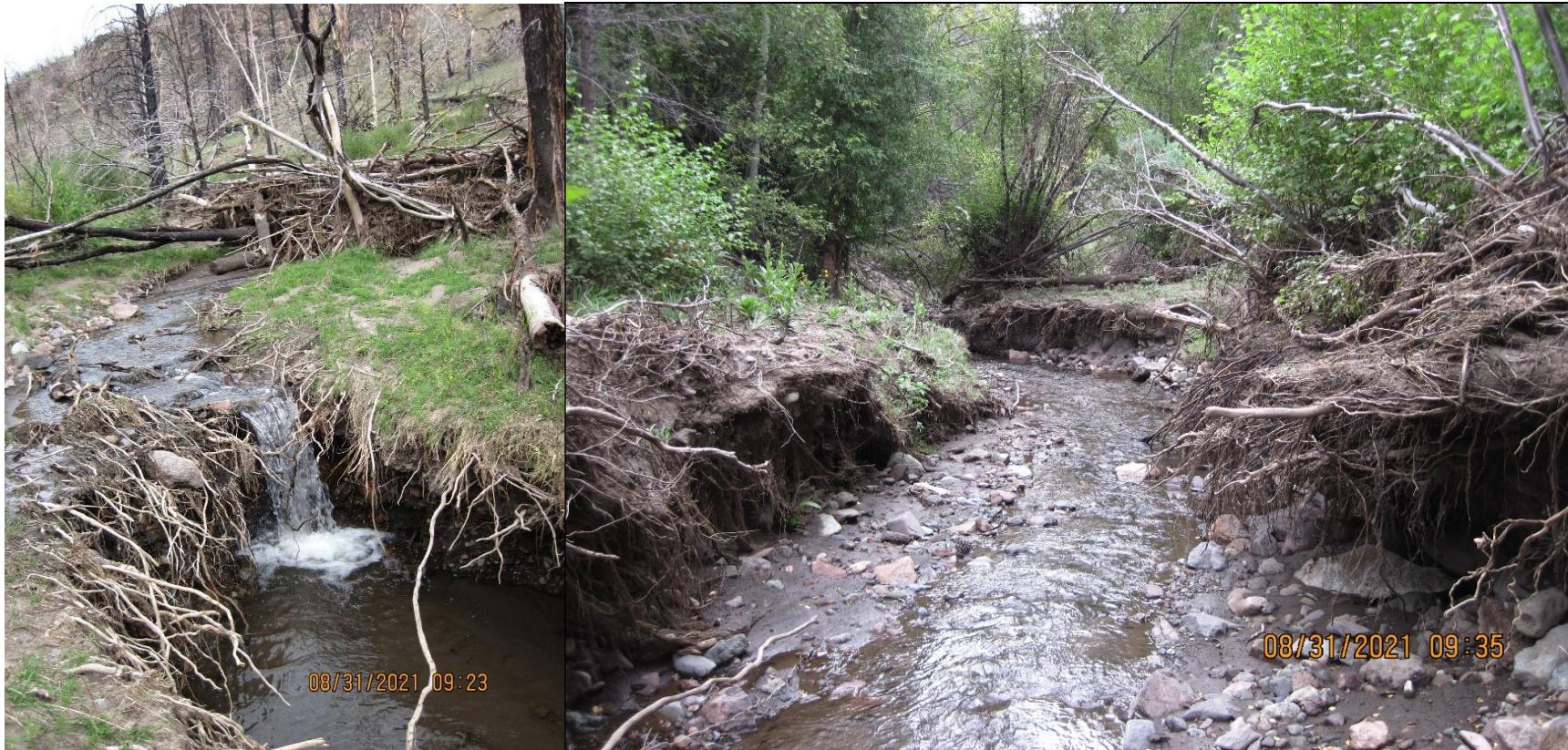
Figure 8. Head cutting, channel incision, and channel widening observed in Threemile Creek in August 2021.
