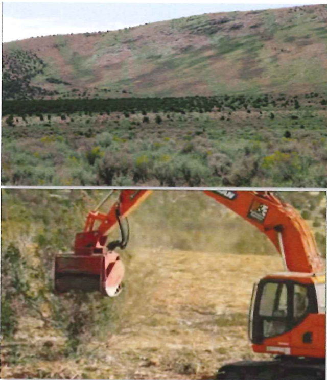
Figure 5 - Higher-density encroachment areas can be managed by using a brush hog to remove conifers.
